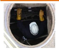
Performing electrical work in confined spaces and enclosed areas including underground electrical vaults, manholes and similar structures can be dangerous and fatal if the work is not done properly. Workers need to have the required training in first aid, CPR, rescue, and communication procedures before they perform tasks inside these spaces.
