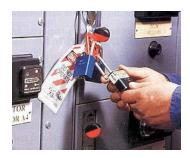
Each worker who works on the machine must lock out and tag the power disconnect. Never assume that the machine you are working on has been disconnected and locked out unless you have done it yourself.
