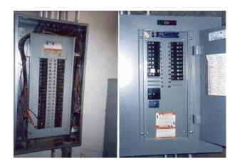
Covers on openings and approved electrical boxes restrict access to the exposed energized parts inside the openings and boxes.
