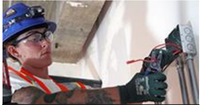
Demi Zayas installs electrical wiring.
