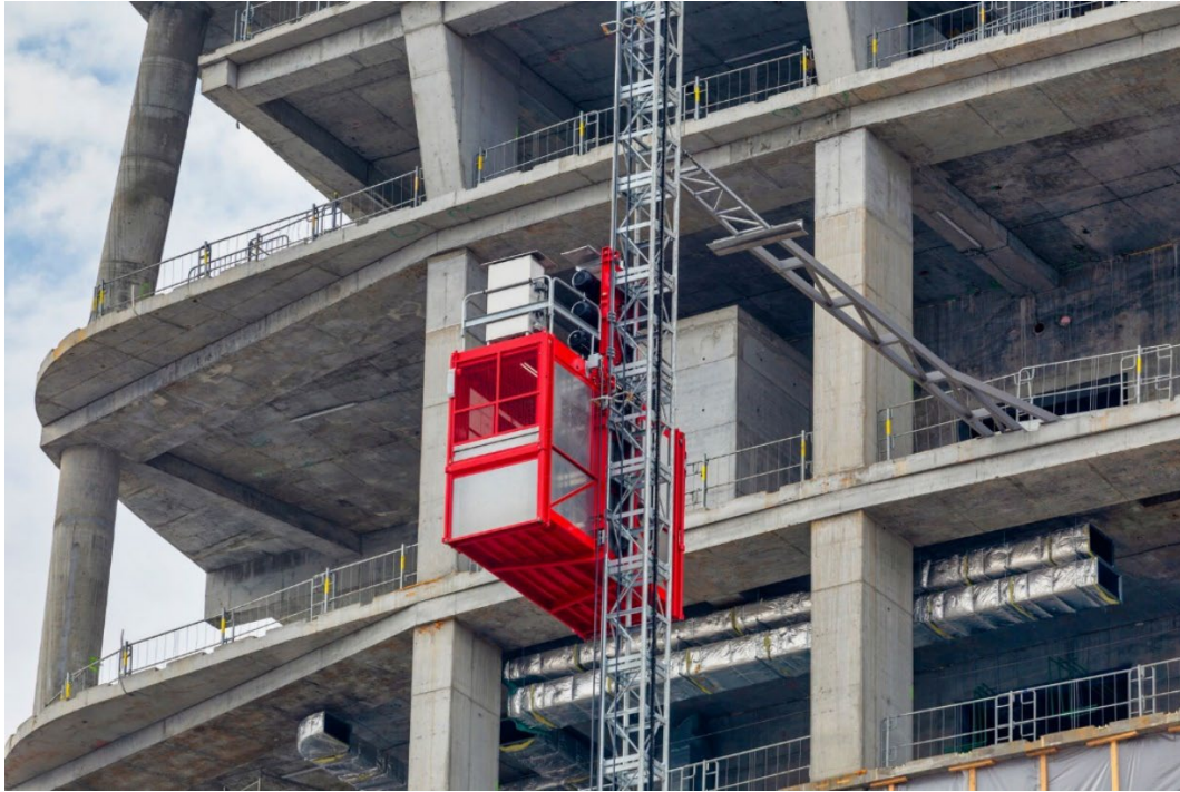
Figure 1. A Construction Personnel Hoist (CPH) is a temporary elevator used for carrying personnel and materials at construction sites. The hoist car in red coloring, consists of a “net platform area” which is the total floor space inside the hoist car. (Photo Credit: Technical Safety BC)
